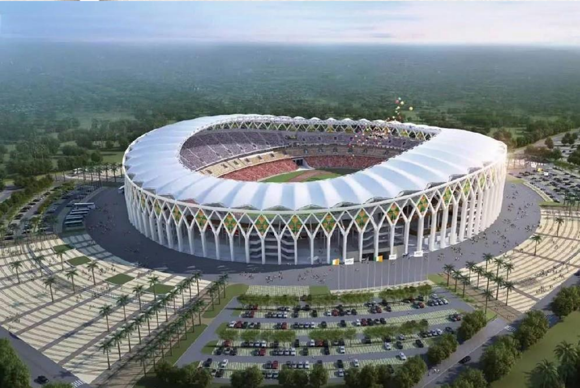
The stadium project in Côte d'Ivoire aided by the Chinese government.
