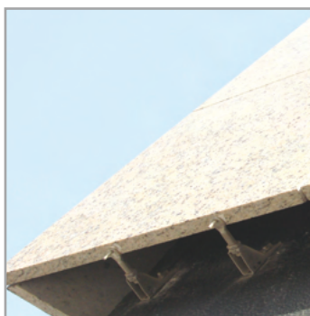
• AXO body anchors are used to install stone panels at horizontal joints to concrete substrate
